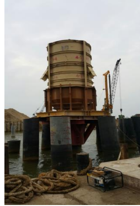
Figure 4: During Preparation of Statnamic Test
