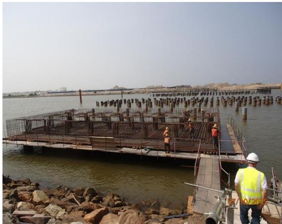
Figure 7: During Preparation for Pile Cap Casting
