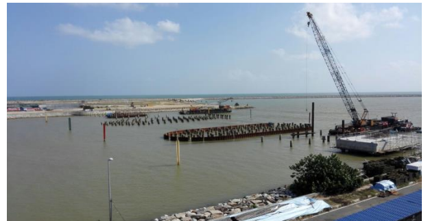
Figure 2: Site Condition during Construction of Pile Cap
