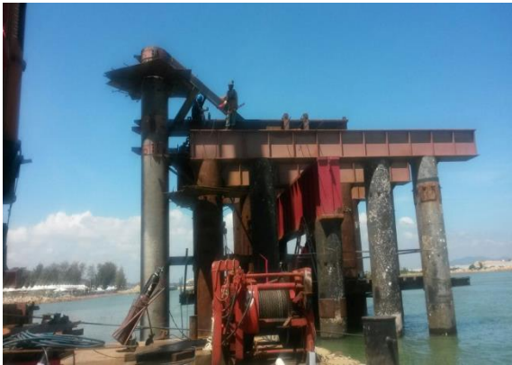
Figure 6: Site Preparation for Lateral Pile Load Test
